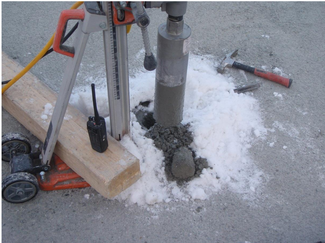
Photo 1: Drilled core attempt near the center of the dam. Melted core prompted a change in placement direction.
