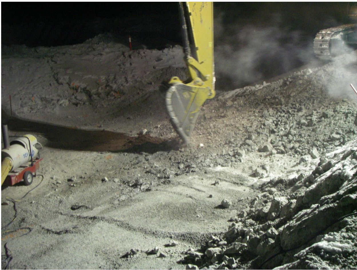
Photo 7: The CAT 345 excavator equipped with tiger teeth is removing the 5/8 crush in the north-east corner of the key-trench.
