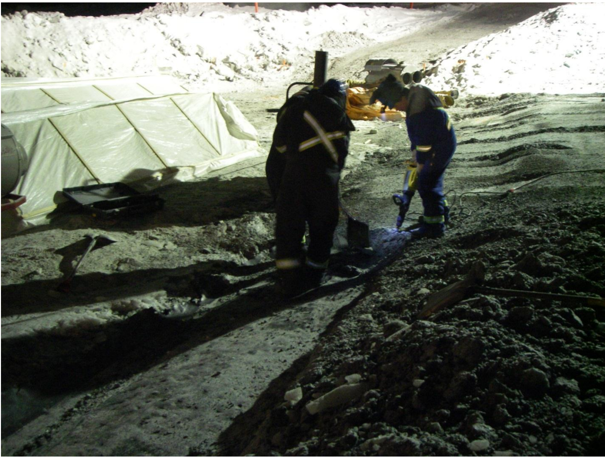
Photo 6: Workers exposing the HDPE liner around Sta. 1+80. A jackhammer was used to loosen up frozen the 5/8 crush. A few holes punched in the HDPE and the underlying GCL by the jackhammer can be seen in the foreground.
