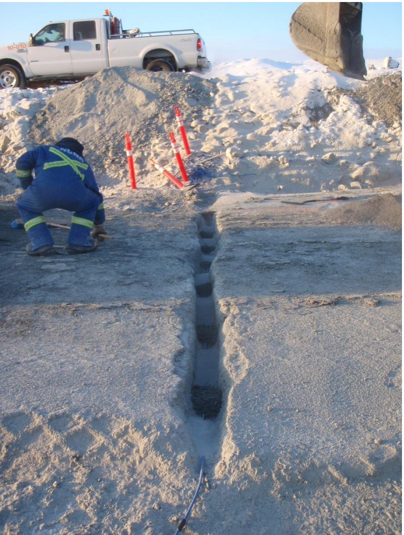
Photo 3: Thermistor string ND-HTS-175-33.5, installed with bentonite powder water stops.
